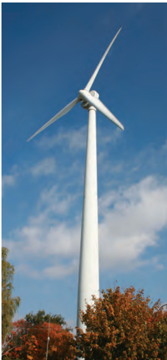
Figure 6.38 The ExPlace wind turbine is 90 m tall to the tip of the blade and has a rotor diameter of 52 m. It has a normal rotation speed of 24.5 revolutions per minute and can generate about 500 kW of electrical power in winds of 11 m/s.
