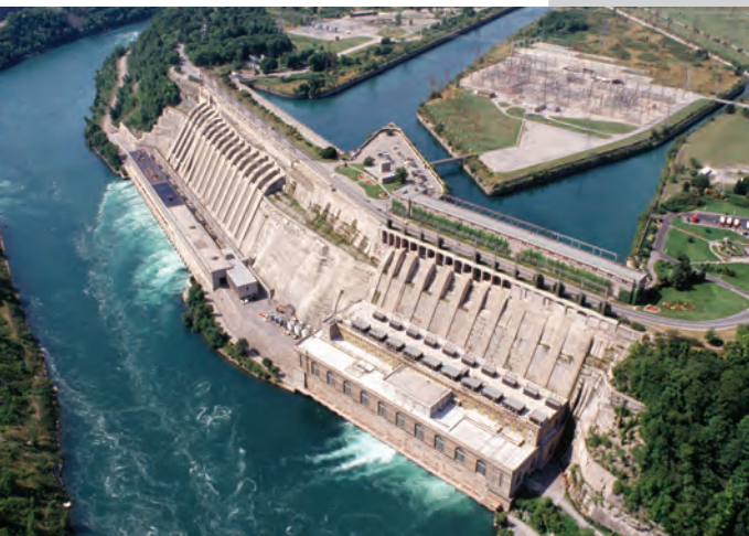
Figure 6.36 A hydroelectric generating plant. The amount of potential energy in water is proportional to the head — the difference in height between the source and the turbine.
