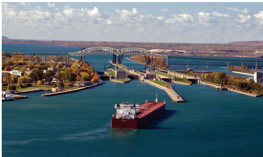
Figure 6.15 A lock raises and lowers boats between stretches of water of different levels. The Soo Locks at Sault Ste. Marie connect Lake Huron to the higher Lake Superior.
