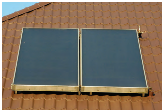
Figure 7.38 Flat-plate collectors are the most common type of solar collectors used in solar water-heating systems in homes.
