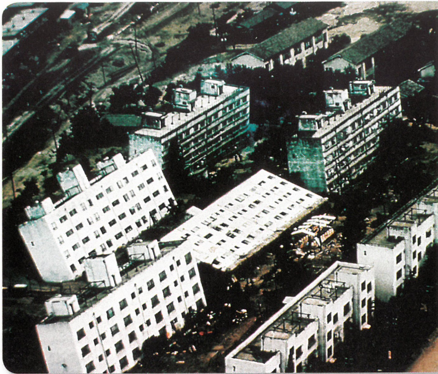
■ Figure 19.22 Soil liquefaction happens when seismic vibrations cause poorly consolidated soil to liquefy and behave like quicksand. The buildings pictured here were built on this type of soil and an earthquake caused the buildings to sink into the ground.
