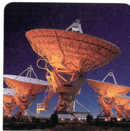
■ Figure 27.5 The Very Large Array is situated near Socorro, New Mexico. The dish antennae of this radio telescope are mounted on tracks so they can be moved to improve resolution.
